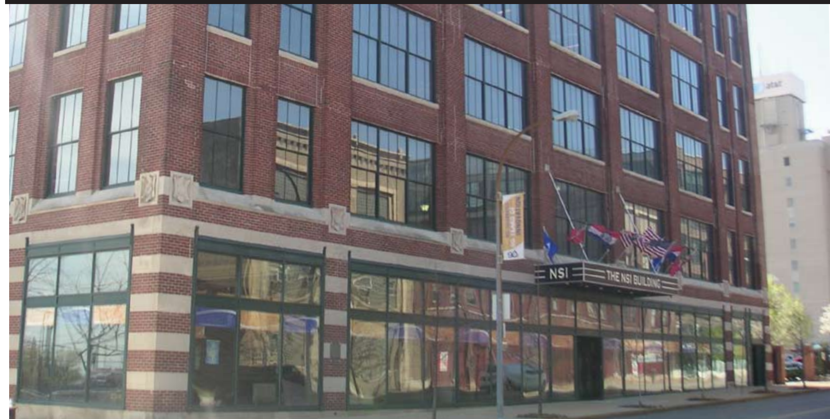
NSI Building at 2300 Locust
